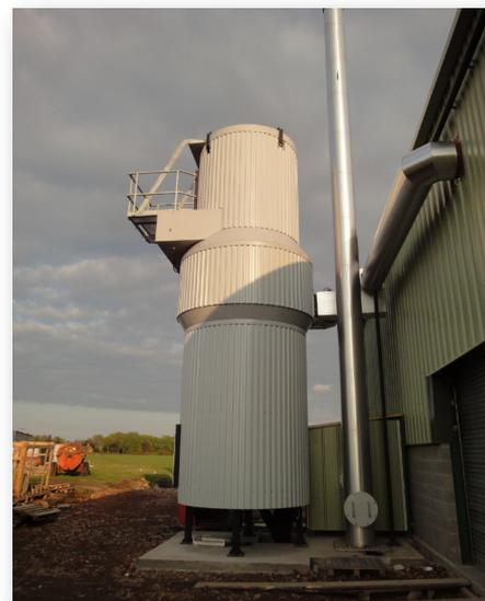
*A biomass boiler bag filter for removing particulates from flue gas*
