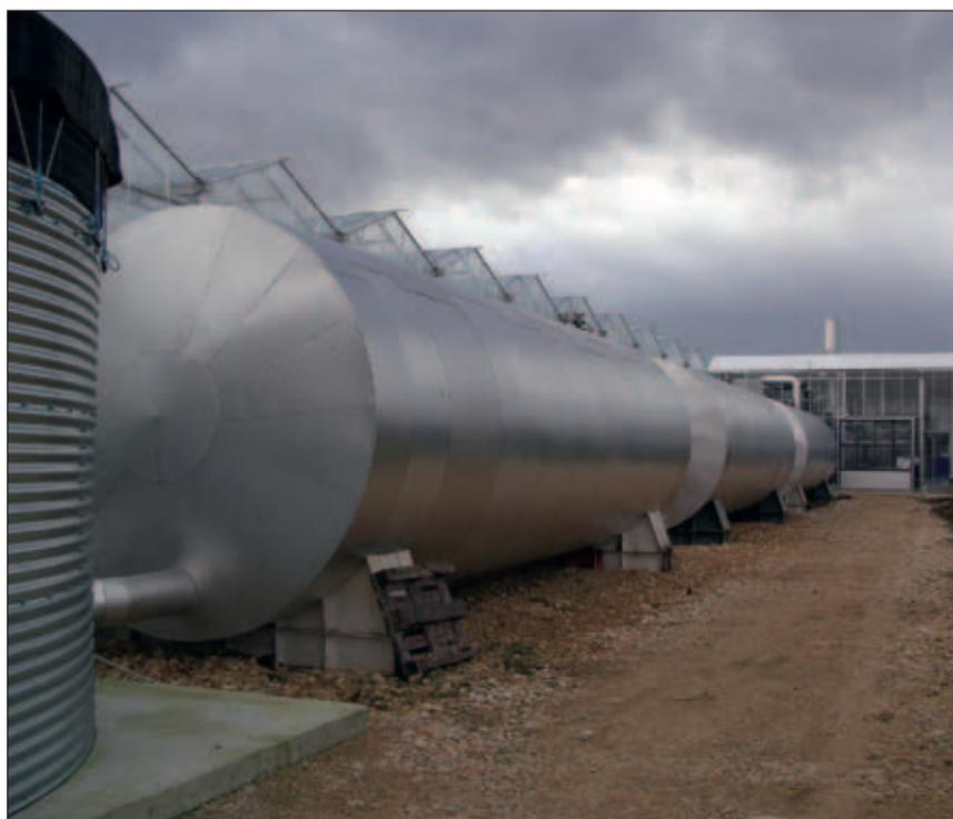
1 Well insulated heat storage tanks are essential to reduce the energy costs of CO<sub>2</sub> enrichment by the burning of fossil fuels
