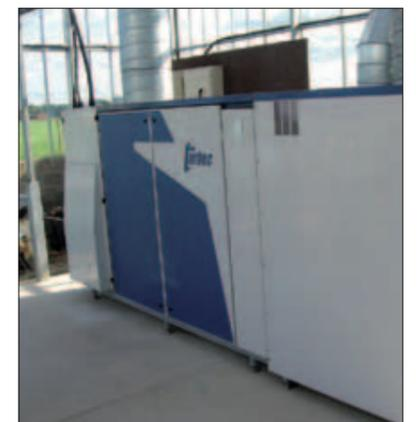
**2 Micro-turbine CHP units can provide CO<sub>2</sub> for glasshouse enrichment without the need for a catalytic converter to remove harmful pollutants**
