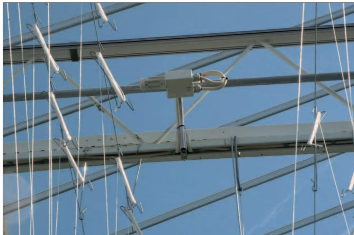
**4** If at all possible: remove the lamp, reflector and electronic luminaire in summer to reduce crop shading
