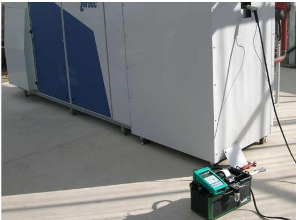
'cleanliness' of the flue gases. It demonstrates that the micro-turbine has 1.5ppm NO<sub>x</sub> to every 10,000ppm of CO<sub>2</sub>; and can therefore be considered as clean burning, especially when compared to the reciprocating engine at 7ppm NO<sub>x</sub> to every 10,000ppm CO<sub>2</sub>. As expected the results from the boilers fall between these two, with the new boiler burning cleaner than the old boiler.
