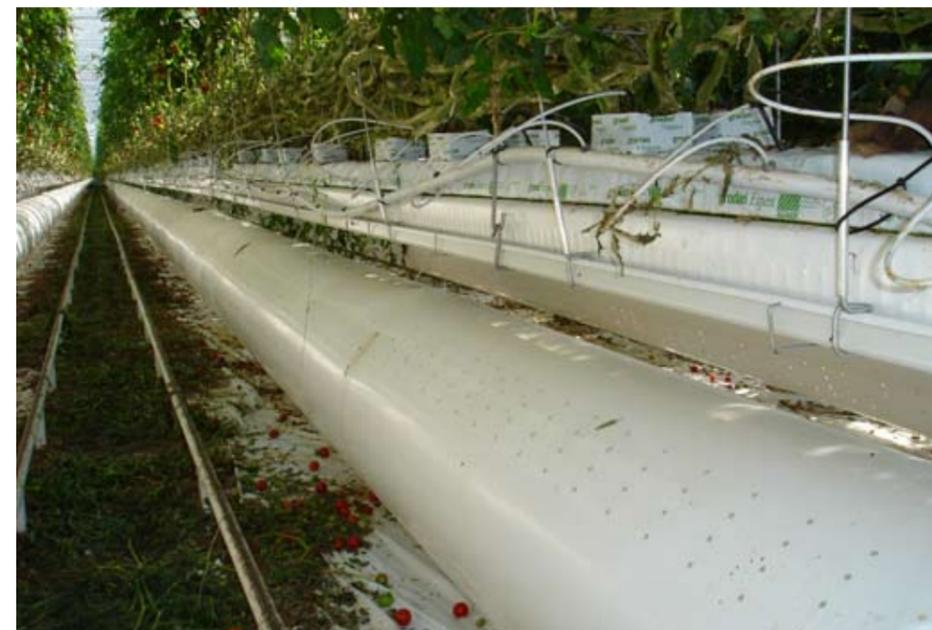
The Dutch systems use underground aquifers for long-term energy storage. Therefore the Mill Nurseries' installation is using heat from their existing boiler and CHP with heating water temperatures being limited to a maximum of 50°C to simulate the use of low grade or waste heat. Also, the Dutch rely on the aquifer to provide cooling energy in the summer. Again this is not viable in the UK so the only cooling provided is from outside air.
